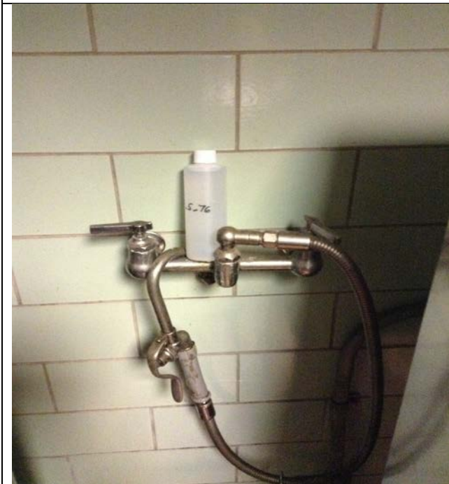
View of Kitchen Spigot Location, Sample #: 448.5-76
